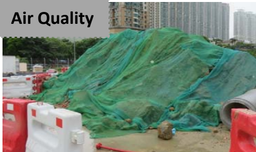
Stockpiles of aggregate covered by tarpaulin to prevent windblown dust.
