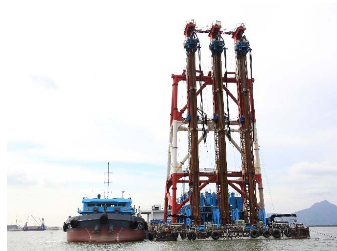
DCM Barge for Marine DCM Installation
