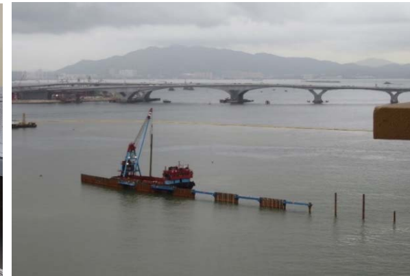
Perimeter silt curtain
