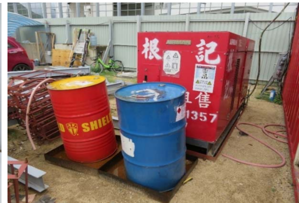
Drip trays for chemical storage
