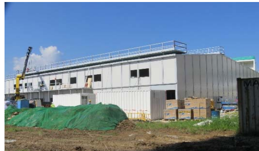
Stockpiles of aggregate covered by tarpaulin to prevent windblown dust.
